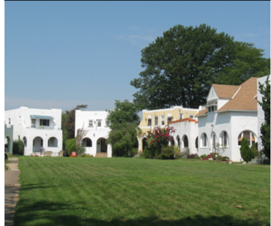
Villa Monterey (Corinne Court), New Castle County
